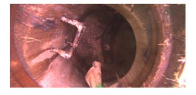
Description: **Deposits Attached Ragging** Distance (ft): .0 Structural Grade: 0 O&M Grade: 2 Clock Start/From: 6 Clock To: 1st Value: 2nd Value: Value Percent: 5.000 Step: NO
