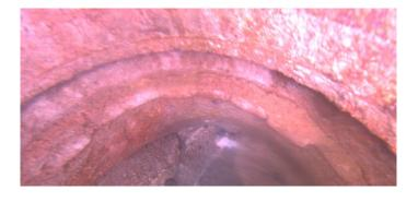
Description: **Deposits Attached Other** Distance (ft): .0 Structural Grade: 0 O&M Grade: 2 Clock Start/From: 12 Clock To: 12 1st Value: 2nd Value: Value Percent: 5.000 NO Step: Remarks: **Mixed materials**
