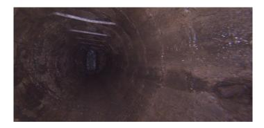
Code: HSV Hole Soil Visible Description: Distance (ft): 3.6 Structural Grade: 5 O&M Grade: 0 Clock Start/From: 3 Clock To: 1st Value: 2nd Value: Value Percent: Step: NO Remarks:
