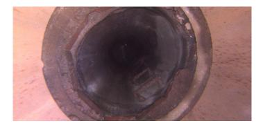
Code: DB Description: **Displaced Brick** Distance (ft): .0 Structural Grade: 3 O&M Grade: 0 Clock Start/From: 4 Clock To: 5 1st Value: 2nd Value: Value Percent: Step: NO
