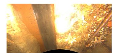
Code: Description: **Deposits Settled Gravel** Distance (ft): 15.3 Structural Grade: 0 O&M Grade: 2 Clock Start/From: 12 Clock To: 12 1st Value: 2nd Value: Value Percent: 5.000 Step: NO Remarks:
