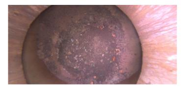
Code: DAZ Description: **Deposits Attached Other** Distance (ft): 1.2 Structural Grade: 0 O&M Grade: 2 Clock Start/From: 12 Clock To: 12 1st Value: 2nd Value: Value Percent: 10.000 Step: NO Remarks: **Mixed materials**
