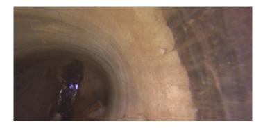
Code: CL Description: Crack Longitudinal Distance (ft): 1.2 Structural Grade: 2
