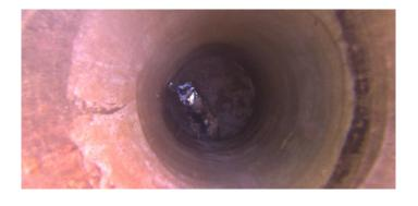
Description: **Crack Longitudinal** Distance (ft): .0 Structural Grade: 2 O&M Grade: 0 Clock Start/From: 9 Clock To: 1st Value: 2nd Value: Value Percent: NO Step:
