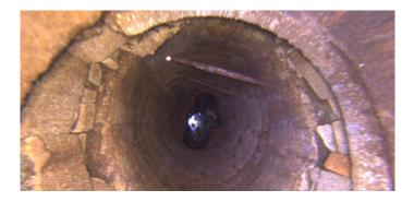
Code: DB Description: **Displaced Brick** Distance (ft): .0 Structural Grade: 3 O&M Grade: 0 Clock Start/From: 8 Clock To: 4 1st Value: 2nd Value: Value Percent: Step: NO Remarks:
