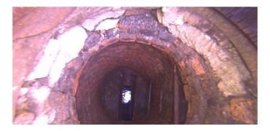
Code: DB Description: **Displaced Brick** Distance (ft): .0 Structural Grade: 3 O&M Grade: 0 Clock Start/From: 9 3 Clock To: 1st Value: 2nd Value: Value Percent: Step: NO Remarks:
