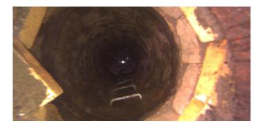
Code: DB Description: **Displaced Brick** Distance (ft): .0 Structural Grade: 3 O&M Grade: 0 Clock Start/From: 12 Clock To: 12 1st Value: 2nd Value: Value Percent: Step: NO Remarks:
