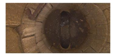
Code: SSS Surface Spalling Description: Distance (ft): 4.4 Structural Grade: 2 O&M Grade: 0 Clock Start/From: 8 Clock To: 9 1st Value: 2nd Value:
