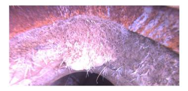
Code: RMJ Description: **Roots Medium Joint** Distance (ft): .0 Structural Grade: 0 O&M Grade: 3 Clock Start/From: 12 Clock To: 12 1st Value: 2nd Value:
