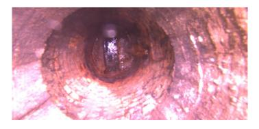
Code:FLDescription:Fracture LongitudinalDistance (ft):.0Structural Grade:3O&M Grade:0Clock Start/From:8Clock To:.11st Value:.22nd Value:.
