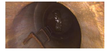
Description: **Surface Roughness Increased** Distance (ft): .0 Structural Grade: 1 O&M Grade: 0 Clock Start/From: 12 Clock To: 12 1st Value: 2nd Value: Value Percent: Step: NO Remarks:
