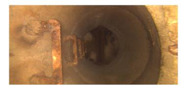
Code: MMC Description: Material Change Distance (ft): 1.5 Structural Grade: 0 O&M Grade: 0 Clock Start/From: Clock To: 1st Value: 2nd Value:
