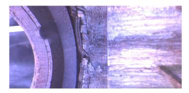
Code: ISSR Intruding Sealing Ring Description: Distance (ft): 1.5 Structural Grade: 0 O&M Grade: 2 Clock Start/From: 9 Clock To: 10 1st Value: 2nd Value: Value Percent: 0.000 Step: NO Remarks:
