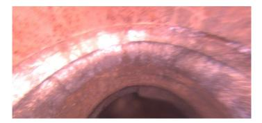
Code: DAZ Description: **Deposits Attached Other** Distance (ft): .4 Structural Grade: 0 O&M Grade: 2 Clock Start/From: 12 Clock To: 12 1st Value: 2nd Value: Value Percent: 5.000 Step: NO Remarks: **Mixed materials**
