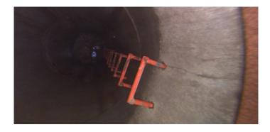
Code: СМ Description: **Crack Multiple** Distance (ft): .7 Structural Grade: 3 O&M Grade: 0 Clock Start/From: 2 3 Clock To: 1st Value: 2nd Value: Value Percent: Step: NO Remarks:
