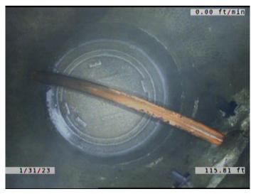
Code: MGO Description: **Miscellaneous General Observation** Distance (ft): 115.8 Structural Grade: 0 0 O&M Grade: Clock Start/From: Clock To: 1st Value: 2nd Value: Value Percent: Continuous Index: Within 8" of Joint: NO Remarks: LOOKS TO BE FIBER OPTIC CROSS BORED THROUGH THE MANHOLE.
