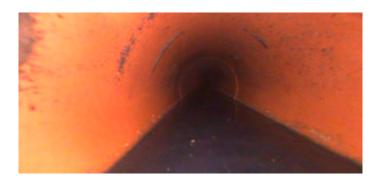
Distance (ft): 13.1 Structural Grade: 0 O&M Grade: 2 Clock Start/From: 7 Clock To: 5
