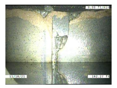
Code: MWLS Description: **Miscellaneous Water Level Sag** Distance (ft): 162.3 Structural Grade: 2 0 O&M Grade: Clock Start/From: Clock To: 1st Value: 2nd Value: Value Percent: 10.000 Continuous Index: F05 Within 8" of Joint: NO Remarks:
