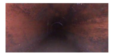
Code:RPRDescription:Repair Point Pipe Replaced
