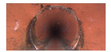
Distance (ft): 89.4 Structural Grade: 0 O&M Grade: 2 Clock Start/From: 8 Clock To: 4 1st Value: 2nd Value: Value Percent: Continuous Index: Within 8" of Joint: YES
