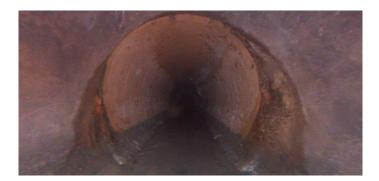
Distance (ft): 3.1 Structural Grade: 0 O&M Grade: 2 Clock Start/From: 7 Clock To: 5
