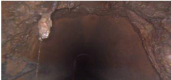
Distance (ft): 3.7 Structural Grade: 0 O&M Grade: 2 Clock Start/From: 8 Clock To: 4
