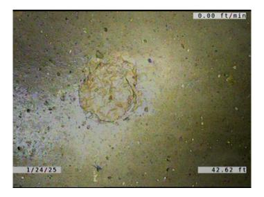
Code: SSC Description: Surface Spalling of Damage Coating 42.6 Distance (ft): Structural Grade: 1 O&M Grade: 0 Clock Start/From: 2 Clock To: 1st Value: 2nd Value: Value Percent: Continuous Index: Within 8" of Joint: YES
