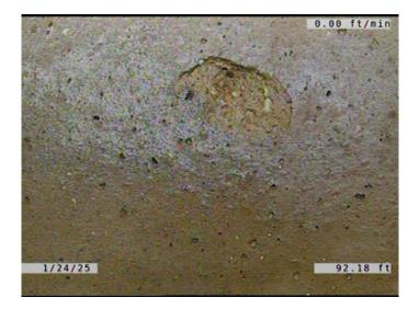
Code: SSC Description: Surface Spalling of Damage Coating Distance (ft): 92.2 Structural Grade: 1 O&M Grade: 0 Clock Start/From: 12 Clock To: 1st Value: 2nd Value: Value Percent: Continuous Index: Within 8" of Joint: YES
