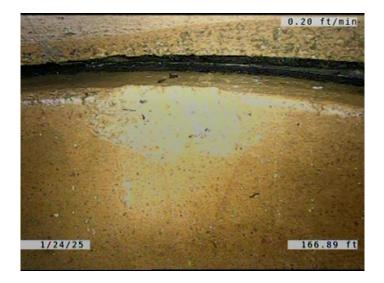
Code: SSS Description: Surface Damage Surface Spalling Distance (ft): 166.9 Structural Grade: 2 O&M Grade: 0 Clock Start/From: 10 Clock To: 1st Value: 2nd Value: Value Percent: Continuous Index: Within 8" of Joint: YES
