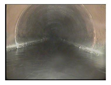
Code: MSA Description: Abandoned Survey Distance (ft): 197.0 Structural Grade: 0 O&M Grade: 0 Clock Start/From: Clock To: 1st Value: 2nd Value: Value Percent: Continuous Index: Within 8" of Joint: NO Remarks: deep sediment
