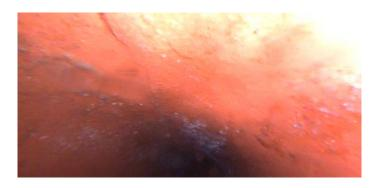
Code: MSA Description: Abandoned Survey Distance (ft): 11.9 Structural Grade: 0 O&M Grade: 0 Clock Start/From: Clock To: 1st Value: 2nd Value: Value Percent: Continuous Index: Within 8" of Joint: NO Remarks: **DEBRIS UNDER WATER**
