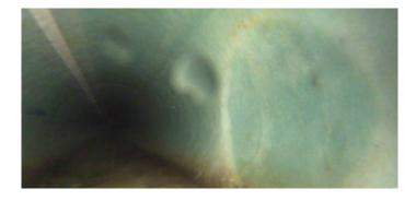
Code: Description: LFAC Lining Failure Abandoned Connection
