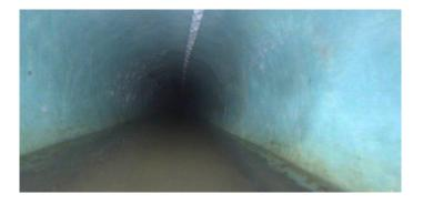
Code: Description: LFAC Lining Failure Abandoned Connection
