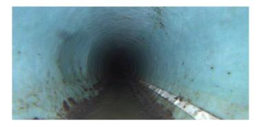
Code: Description: LFAC Lining Failure Abandoned Connection
