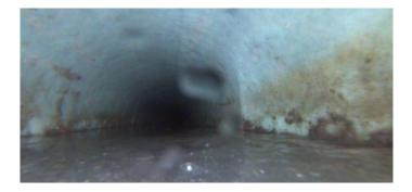
Code: Description: LFAC Lining Failure Abandoned Connection
