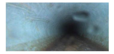
Code:LFWDescription:Lining Failure Wrinkled
