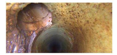
Code: TBD Description: **Tap Break-in Defective** Distance (ft): 26.4 Structural Grade: 0 O&M Grade: 3 Clock Start/From: 11 Clock To: 1st Value: 4.000 2nd Value: Value Percent: Continuous Index: Within 8" of Joint: Remarks: dae
