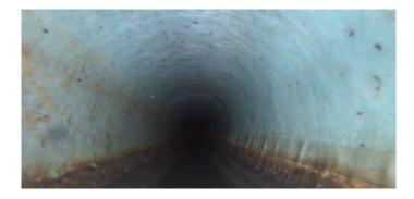
Code: LFAC Description: Lining Failure Abandoned Connection Distance (ft): 9.8 Structural Grade: 0 O&M Grade: 0 Clock Start/From: 3 Clock To: 1st Value: 2nd Value: Value Percent: Continuous Index: Within 8" of Joint: NO Remarks:
