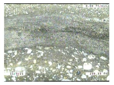
Code: JOMD Description: Joint Offset Medium Defective Distance (ft): 235.3 Structural Grade: 3 O&M Grade: 0 Clock Start/From: Clock To: 1st Value: 2nd Value: Value Percent: Continuous Index: Within 8" of Joint: NO Remarks:
