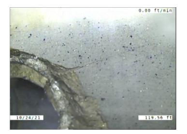
Code: SSS Description: Surface Damage Surface Spalling Distance (ft): 119.6
