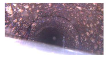
Code: MSA Description: Abandoned Survey Distance (ft): 61.2 Structural Grade: 0 O&M Grade: 0 Clock Start/From: Clock To: 1st Value: 2nd Value: Value Percent: Continuous Index: Within 8" of Joint: NO Remarks: Debris under water
