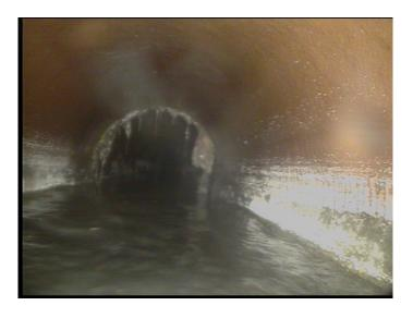
Code: MSA Description: Abandoned Survey 87.0 Distance (ft): Structural Grade: 0 O&M Grade: 0 Clock Start/From: Clock To: 1st Value: 2nd Value: Value Percent: Continuous Index: Within 8" of Joint: NO Remarks: under water debris
