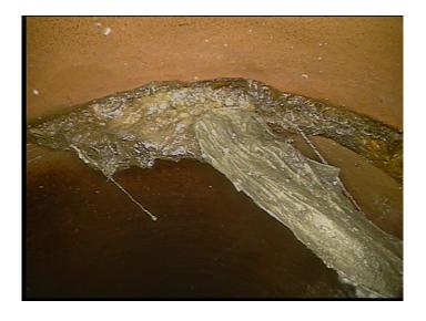
Code: DAE Description: **Deposits Attached Encrustation** Distance (ft): 146.7 Structural Grade: 0 O&M Grade: 2 Clock Start/From: 1 Clock To: 4 1st Value: 2nd Value: 5.000 Value Percent:
