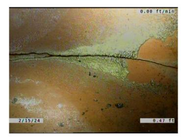
Code: DAE Description: **Deposits Attached Encrustation** Distance (ft): .5 Structural Grade: 0 O&M Grade: 2 Clock Start/From: 3 5 Clock To: 1st Value: 2nd Value: Value Percent: 5.000 Continuous Index: Within 8" of Joint: YES
