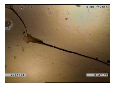
Code: Description: Broken Distance (ft): .5 Structural Grade: 4 0 O&M Grade: Clock Start/From: 9 Clock To: 3 1st Value: 2nd Value: Value Percent: Continuous Index:
