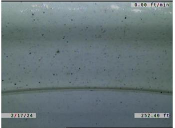
Code: MGO Description: **Miscellaneous General Observation** Distance (ft): 252.4 Structural Grade: 0 0 O&M Grade: Clock Start/From: Clock To: 1st Value: 2nd Value: Value Percent: Continuous Index: Within 8" of Joint: NO Remarks: JOINT/ PIPES NOT PUSHED ALL THE WAY TOGETHER WHEN INSTALLED
