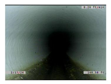
Code: MWLS Description: **Miscellaneous Water Level Sag** Distance (ft): 148.6 Structural Grade: 2 O&M Grade: 0 Clock Start/From: Clock To: 1st Value: 2nd Value: 5.000 Value Percent: Continuous Index: F12 Within 8" of Joint: NO
