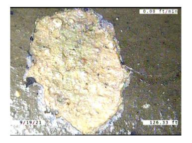
Code: SSS Description: Surface Damage Surface Spalling Distance (ft): 126.3 Structural Grade: 2 O&M Grade: 0 Clock Start/From: 4 Clock To: 7 1st Value: 2nd Value: Value Percent: Continuous Index:
