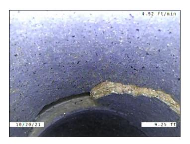
Code: В Description: Broken Distance (ft): 9.3 Structural Grade: 4 O&M Grade: 0 Clock Start/From: 12 Clock To: 2 1st Value: 2nd Value: Value Percent: Continuous Index: Within 8" of Joint: YES
