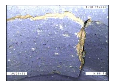
Code: Description: Broken Distance (ft): 5.9 Structural Grade: 4 O&M Grade: 0 Clock Start/From: 11 Clock To: 1 1st Value: 2nd Value: Value Percent: Continuous Index: Within 8" of Joint: YES
