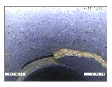
Code: В Description: Broken Distance (ft): 9.3 Structural Grade: 4 O&M Grade: 0 Clock Start/From: 12 2 Clock To: 1st Value: 2nd Value: Value Percent: Continuous Index: Within 8" of Joint: YES
