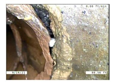
Code: SSS Description: Surface Damage Surface Spalling Distance (ft): 80.6 Structural Grade: 2 O&M Grade: 0 Clock Start/From: 1 3 Clock To: 1st Value: 2nd Value:
