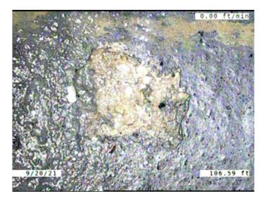
Code: SSS Description: Surface Damage Surface Spalling Distance (ft): 106.6 Structural Grade: 2 O&M Grade: 0 Clock Start/From: 3 Clock To: 1st Value: 2nd Value: Value Percent: Continuous Index: Within 8" of Joint: YES
