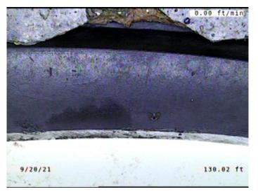
Code: MMC Description: **Miscellaneous Material Change** Distance (ft): 130.0 Structural Grade: 0 O&M Grade: 0 Clock Start/From: Clock To: 1st Value: 2nd Value: Value Percent: Continuous Index: Within 8" of Joint: NO VCP TO PVC Remarks:
