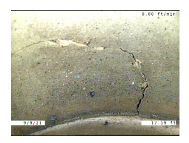
Distance (ft): 17.2 Structural Grade: 4 0 O&M Grade: Clock Start/From: 7 Clock To: 5 1st Value: 2nd Value: Value Percent: Continuous Index: Within 8" of Joint: YES
